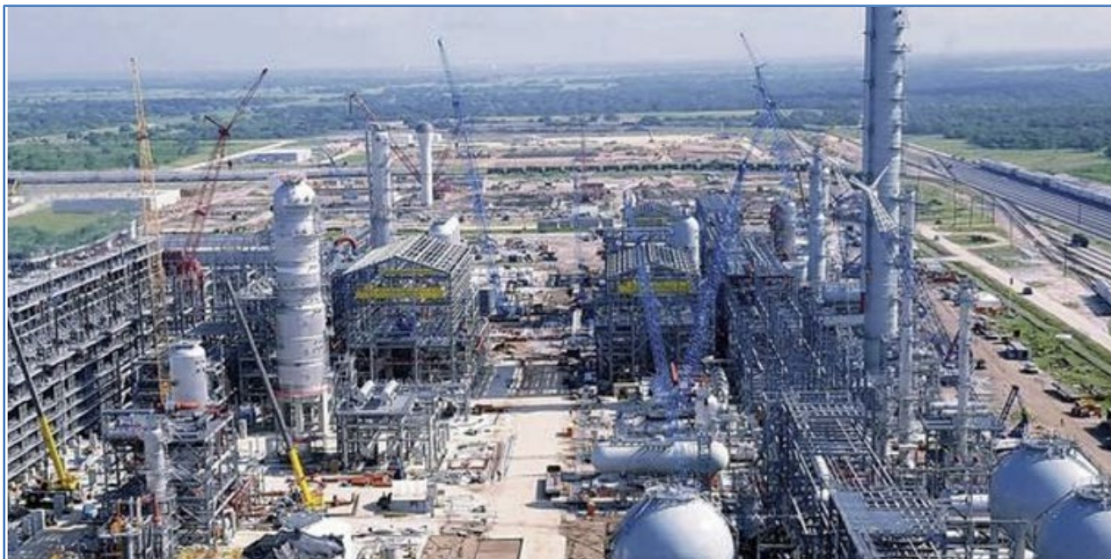
Figure 36 – Formosa's Plant Facilities Undergoing Construction
